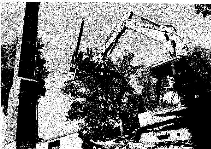
A two-story house on the Farm Creek property in Rowayton is demolished Monday.
